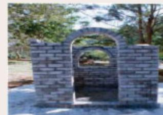
**Bricks made from fly ash**
